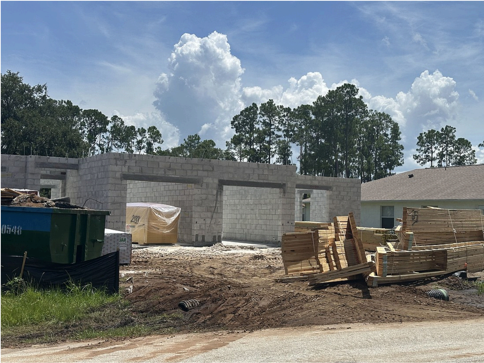
A home under construction in Palm Coast. Photo by Rich Carroll
