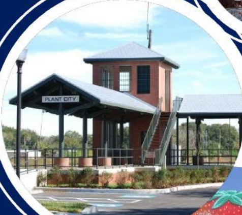
Train Viewing Platform
